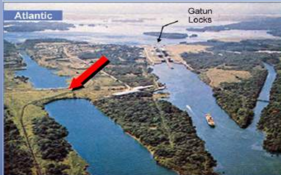
Aerial View of the Construction Sites of the New Locks
